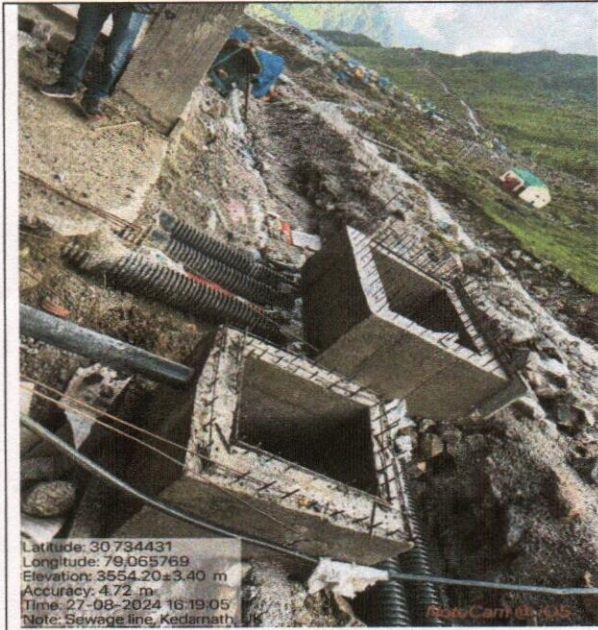
Pic.-5: Construction of sewage lines
